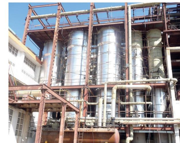
for clear juice, juice circulation and thick juice are also installed. These pumps ensure that the evaporators are supplied with the required amount of juice for concentration. For better heat
