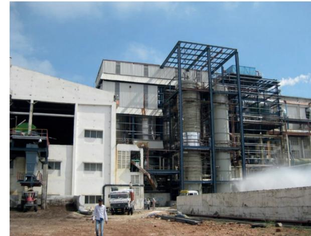
With this upgrade of the evaporation plant, together with optimisation measures in the sugar house, even VP 4 could be used for crystallisation (Figure 5). This raised the factory's processing capacity to 9,000 tcd, and steam consumption was reduced to 28% on cane (without accounting for downtimes) (Figure 6).
