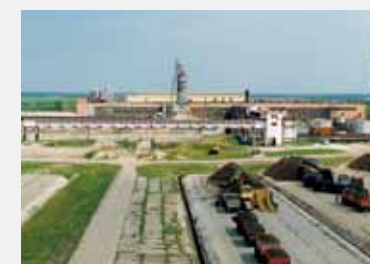
2014-2015: Znamenka, Russia Planning, supply and commissioning of a VKT and automation system; overall planning and project coordination.
